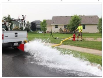
The City of Milaca's annual flushing of fire hydrants removes minerals and sediment that build up over time and ensures that all fire hydrants are in good working order.
