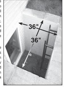
Replacement windows installed in buildings meeting the scope of the International Residential Code shall be exempt from the requirements of Sections R310.1, R310.1.1, R310.1.2, and R310.1.3 if the replacement window meets the following conditions:
