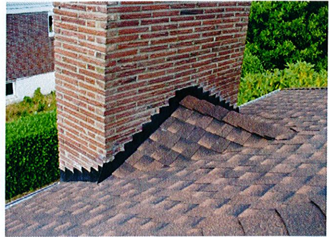
Cricket or saddle at chimney.
